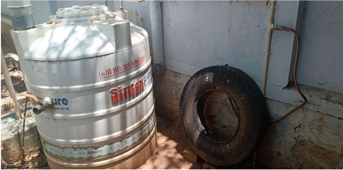
Fig 25: Collected Food waste is dumped in biogas plant and gas is stored in tyre tubes.
